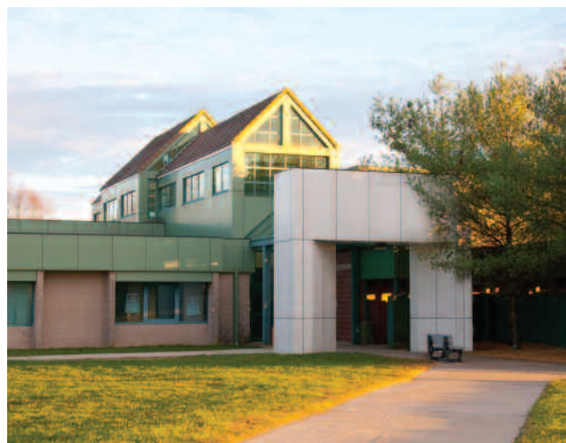
Major roof repairs have been completed college-wide.
