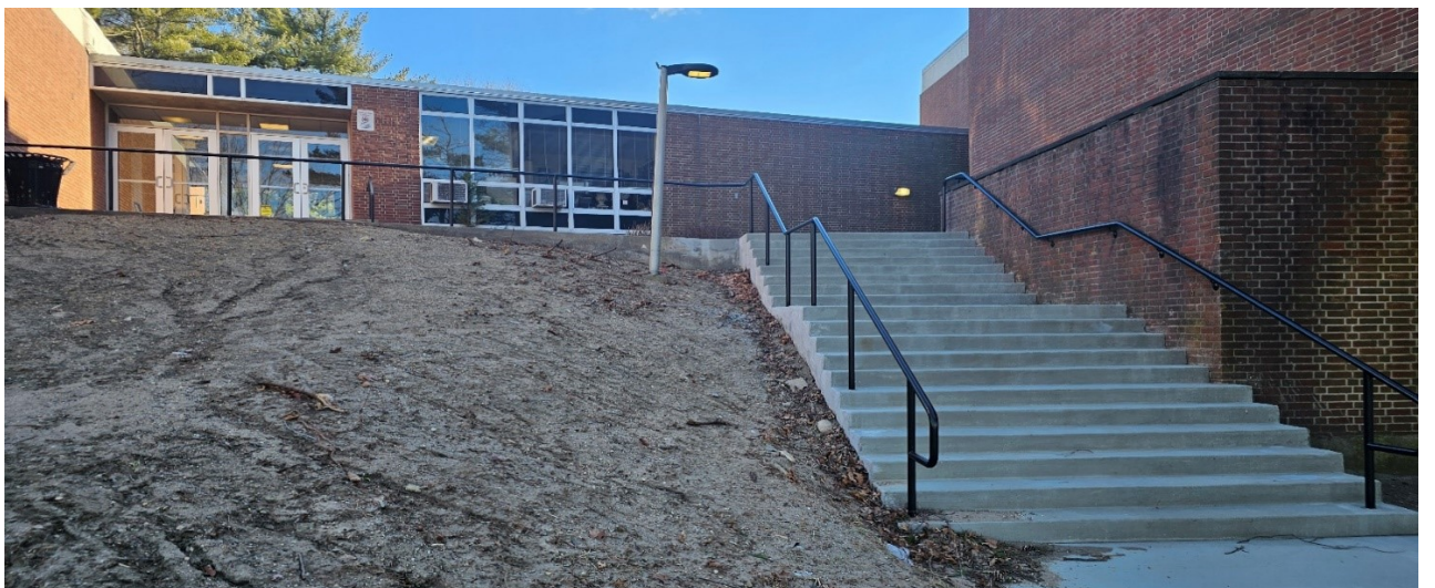
Islip Arts Theater Entrance Staircase Renovation
