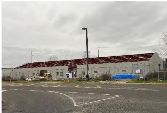
Grant Campus Plant Operations Building
