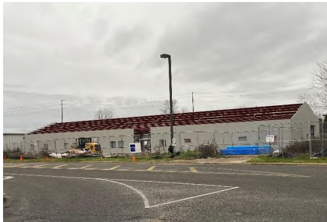
Grant Campus Plant Operations Building
