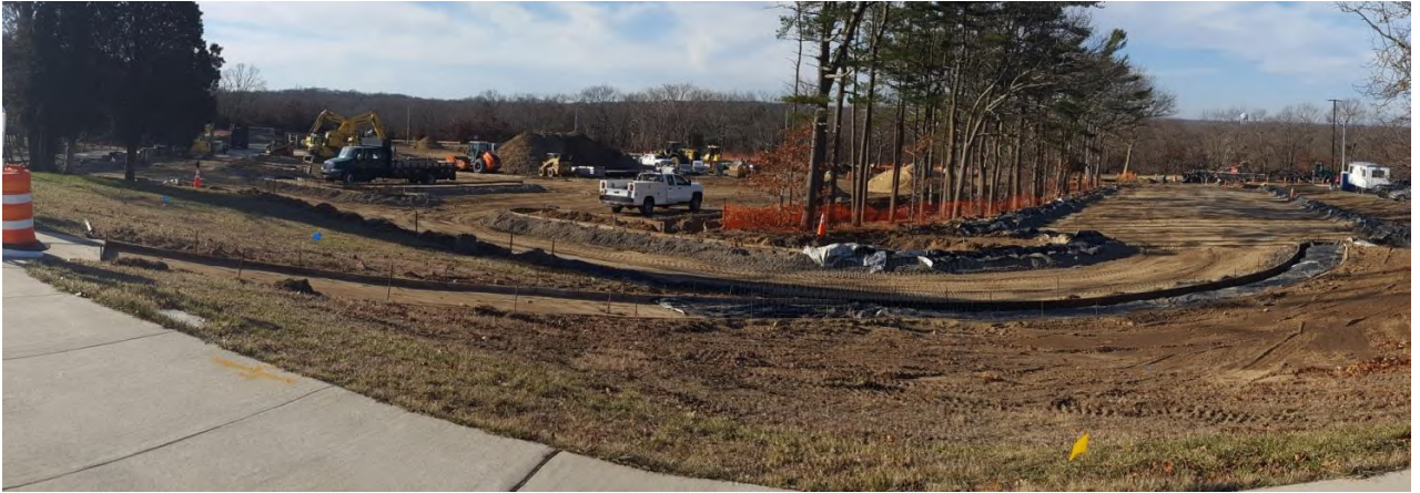
Ammerman Campus - Parking Upgrades
