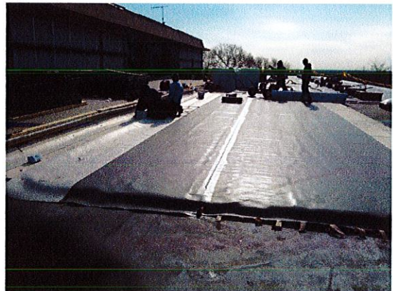
Ammerman Campus Roof Replacements
