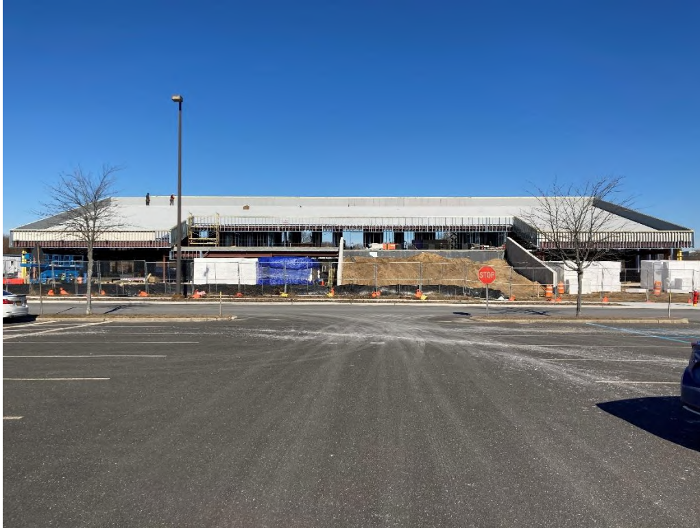
Grant Campus Renewable Energy and STEM Center
